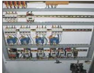
Wiring and final assembly
